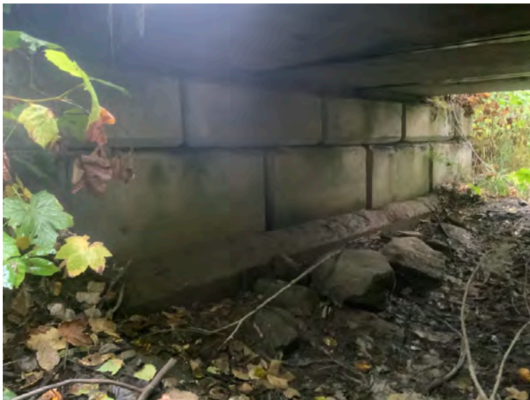
Left Bank Abutment when facing downstream
