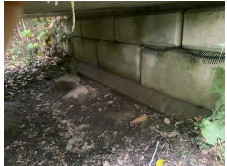
Left Bank Abutment when facing downstream
