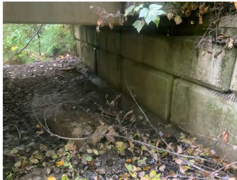
Right Bank Abutment when facing downstream
