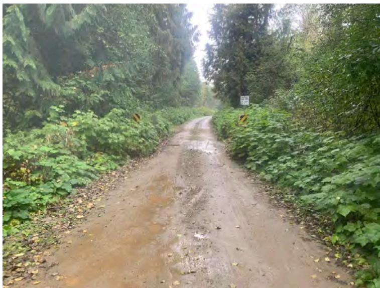
Approach from Right Bank when facing downstream
